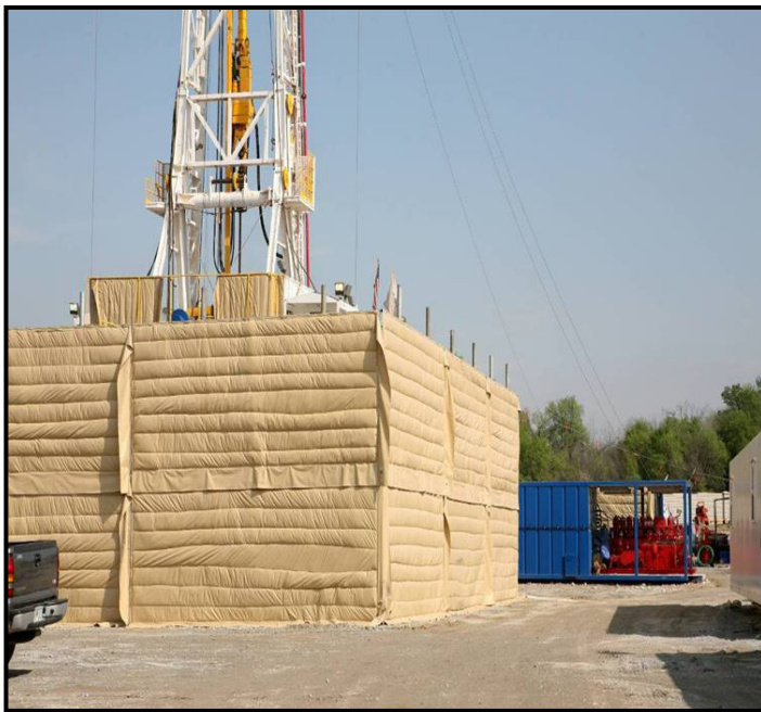
Source : Chesapeake Energy Corporation, 2008 Insulation Blankets Used to Deaden Noise from Drilling Operations
